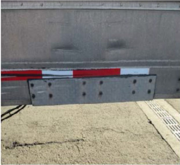
Fig. 2.16 Improper Repair—bolted patch
