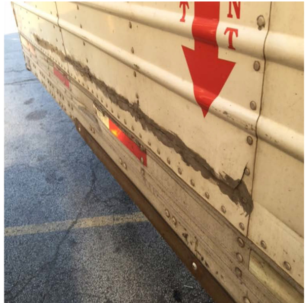
Fig. 2.28 Side panel breaks/cracks
