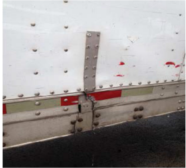
Fig. 2.17 Improper section repair
