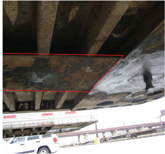
Fig. 3.4 Anti-hook plate—side view
