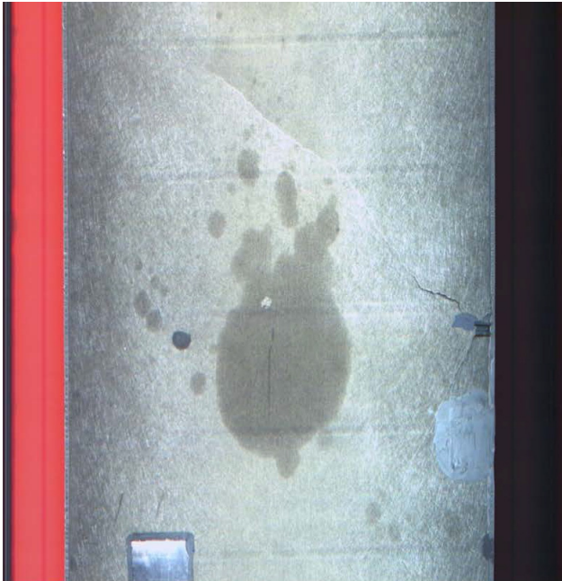
Fig. 2.38 Roof sheet—flex crack
