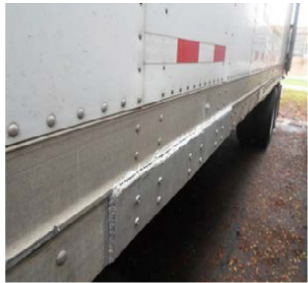
Fig. 2.15 Improper repair—welded patch
