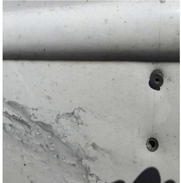
Fig. 2.32 Side panel securement defect
